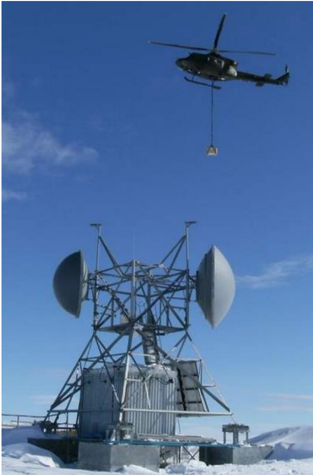
Figure 4. A CH-146 Griffon helicopter slings a battery over a repeater site.
